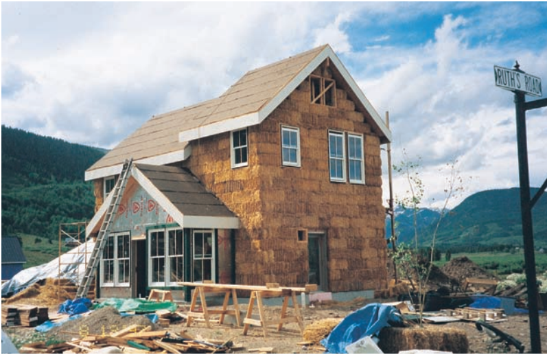
Photo 10 Energy efficient straw bale house in Crested Butte, Colorado (USA) during construction.
