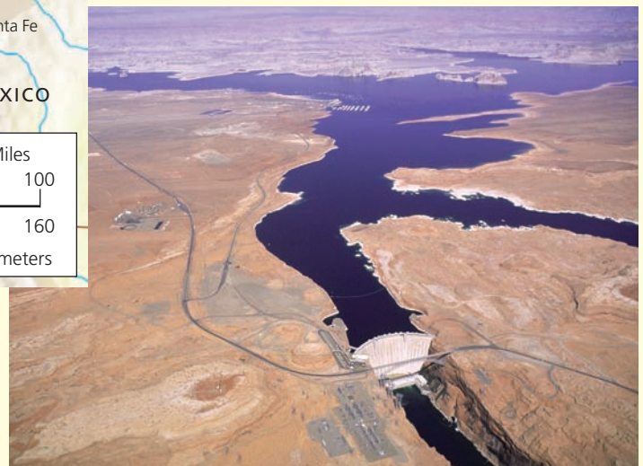
Figure 11-2 Aerial view of Glen Canyon Dam, built across the Colorado River in 1963, and its reservoir, Lake Powell, the second largest reservoir in the United States.
