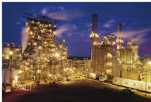
Figure 13-3 Science: refining crude oil. Components of petroleum are removed at various levels, depending on their boiling points, in a giant distillation column. The most volatile components with the lowest boiling points are removed at the top of the column. The photo shows an oil refinery in U.S. state of Texas.
