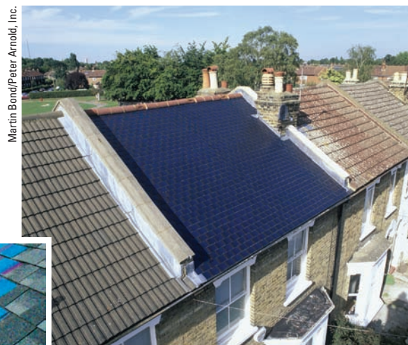
Figure 13-29 Solutions: Photovoltaic (PV) or solar cells can provide electricity for a house or building using solar-cell roof shingles, as shown in this house in Richmond Surrey, England. Solar-cell roof systems that look like a metal roof are also available. In addition, new thin-film solar cells can be applied to windows and outside walls.
