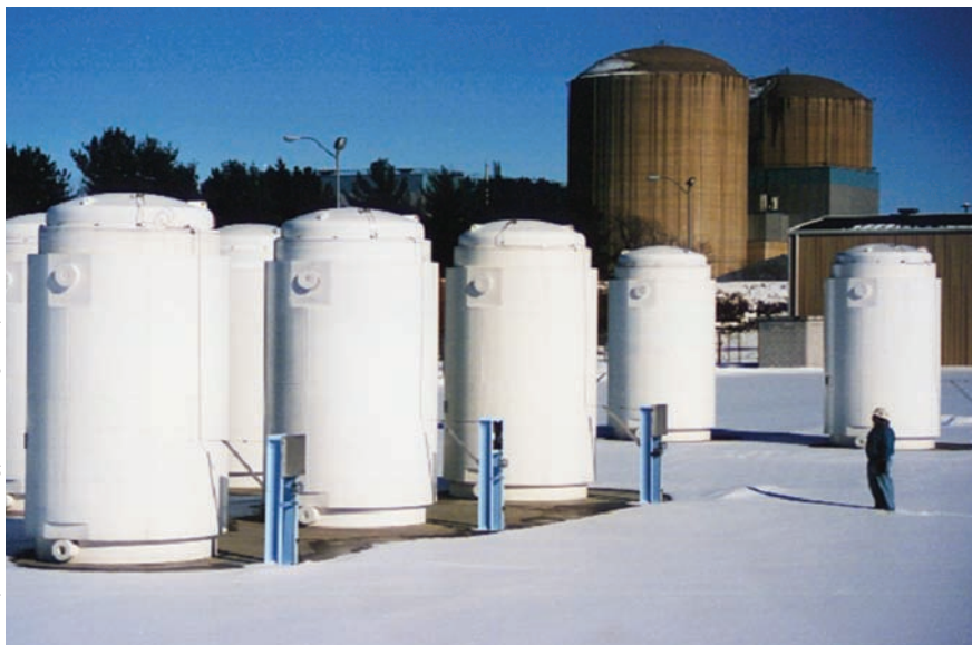
Figure 13-15 Science: after 3 or 4 years in a reactor, spent fuel rods are removed and stored in a deep pool of water contained in a steel-lined concrete basin (left). After they have cooled considerably, some fuel rods are stored upright on concrete pads (right) in dry-storage containers made of steel or concrete. Questions: Do you think these are safe storage methods? Why or why not?
